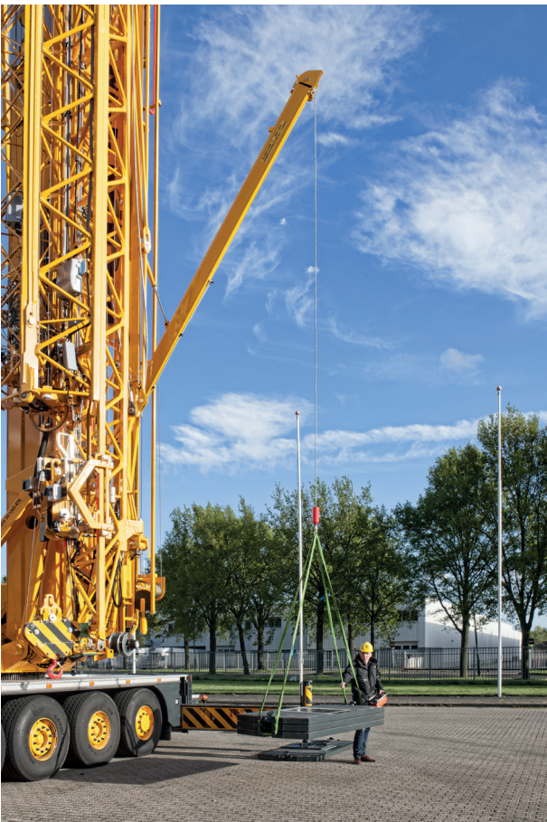
Auxiliary crane for placing the steel pads
